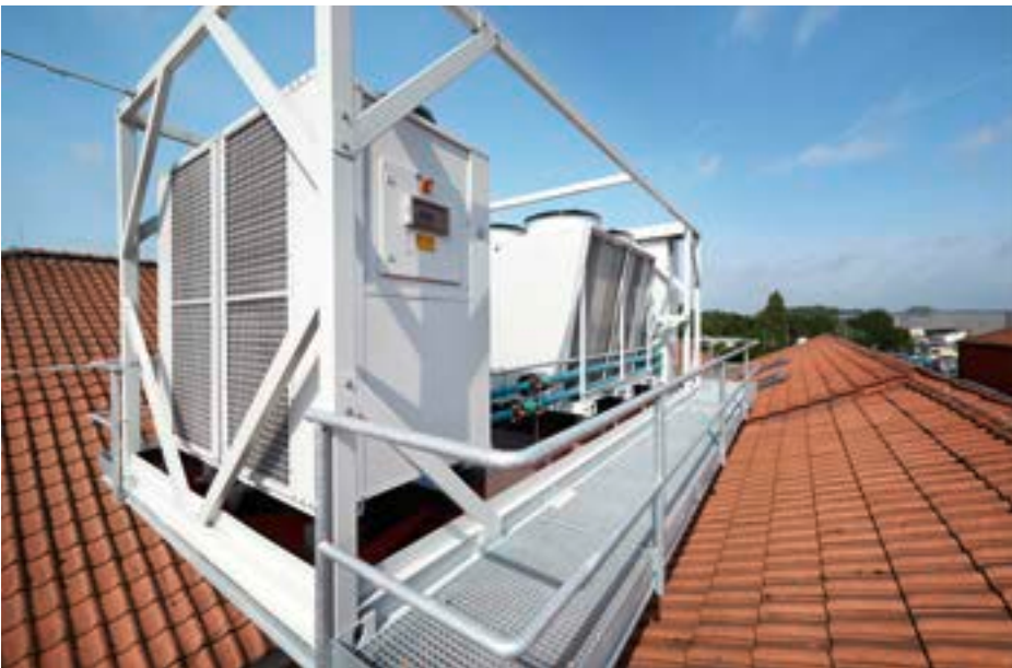
A free cooling system – such as the rooftop chiller shown here – is an easy option that quickly pays off.
